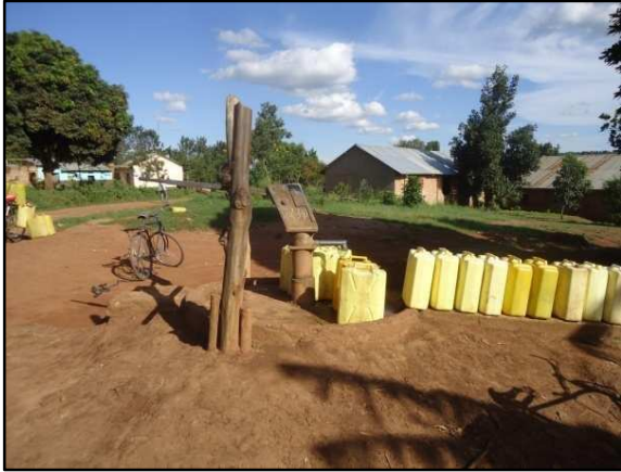
Figure 1-4: A borehole in Mateete Central Parish
