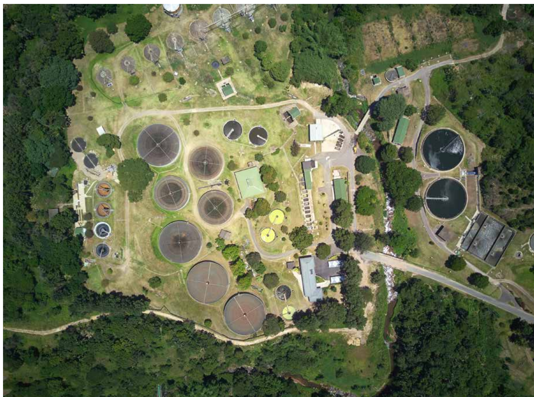
Waste stabilization ponds are designed to remove organic matter and pathogens from wastewater
