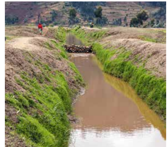
Storm water drainage is a key part of wastewater management
