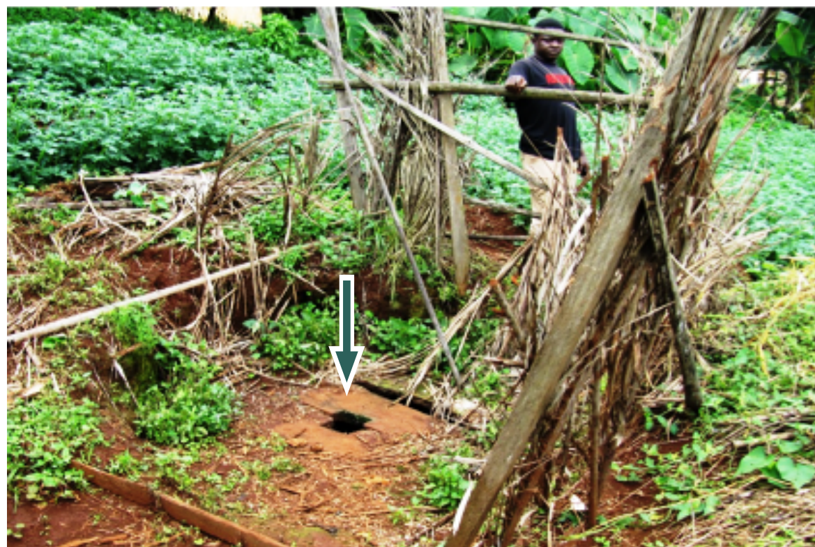
Example of an unimproved pit latrine (see arrow) in Bambui, Northwestern Cameroon.
